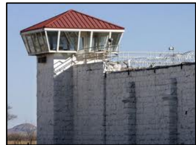
Fig. 2: The Oklahoma State Reformatory was originally built by inmates using granite quarried at nearby Granite Mountain. It houses about 1,000 inmates, most at medium security.
