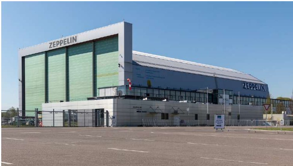
At left: A completed zeppelin hangar of the kind the Port Authority for the State of Minnesota hopes to build next to Little Grandopolis.
