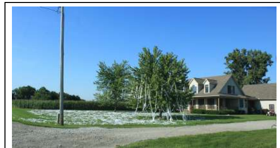
FIG. 5: The GIS campus pre-clean-up.
